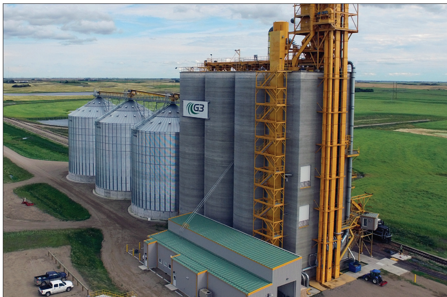
Within three years' time, Grain handler G3 Canada Limited will operate 25 loop-track facilities across Canada, including this one, located in Colonsay, SK.
